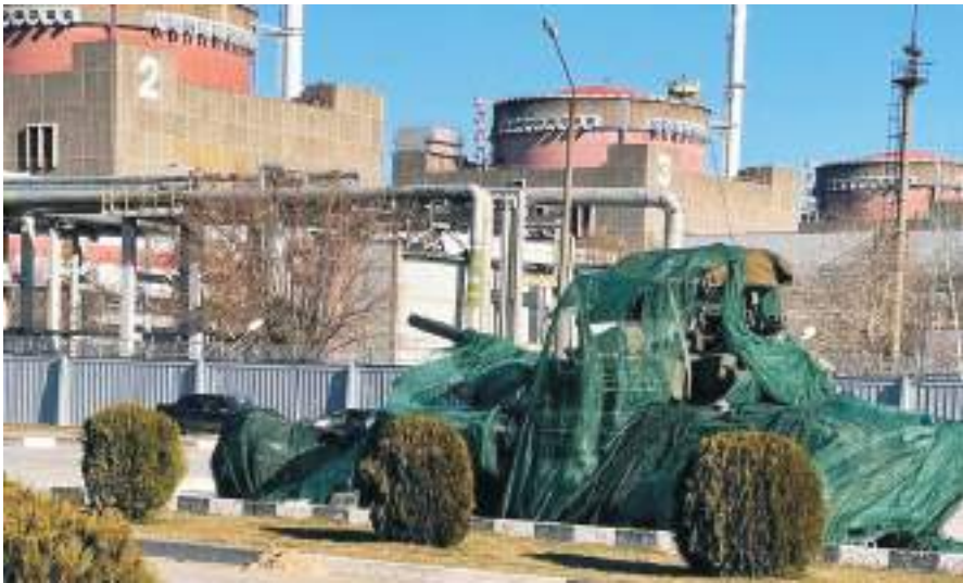
A covered Russian tank outside the Zaporizhzhia nuclear power plant
