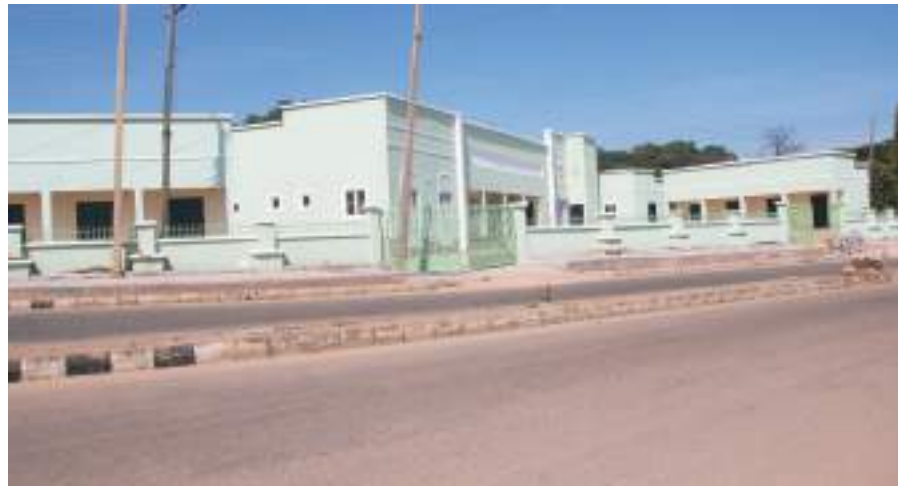
Front view of the remodeled NUJ State Secretariat
