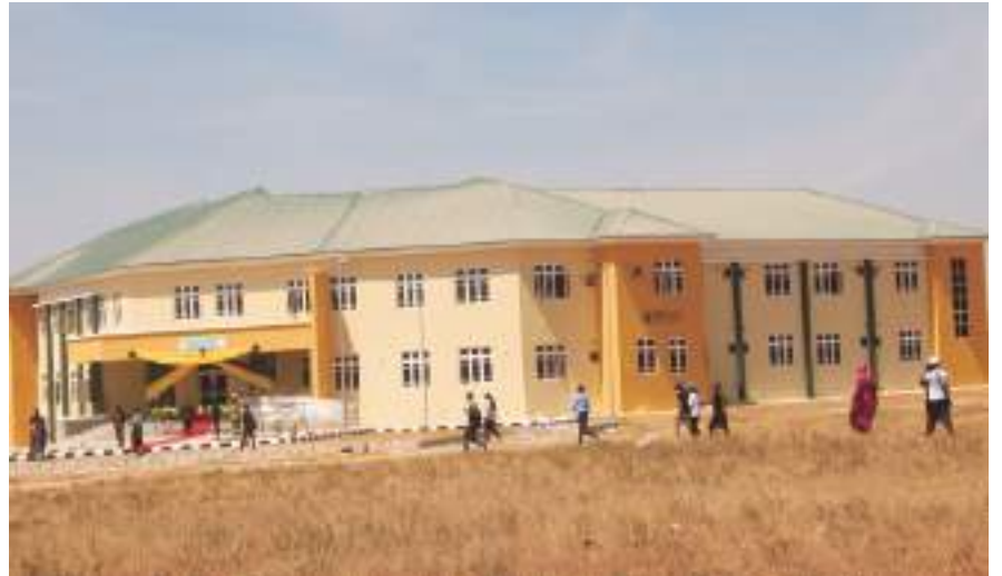
Project commissioned during the 6th and 7th PLASU convocation
