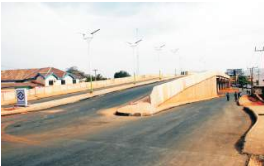
Photo showing the flyover from Dogon Karfe to Terminus and Lamingo road junction roundabout
