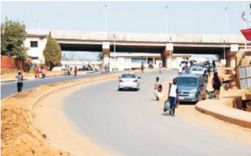
Front view of the flyover
