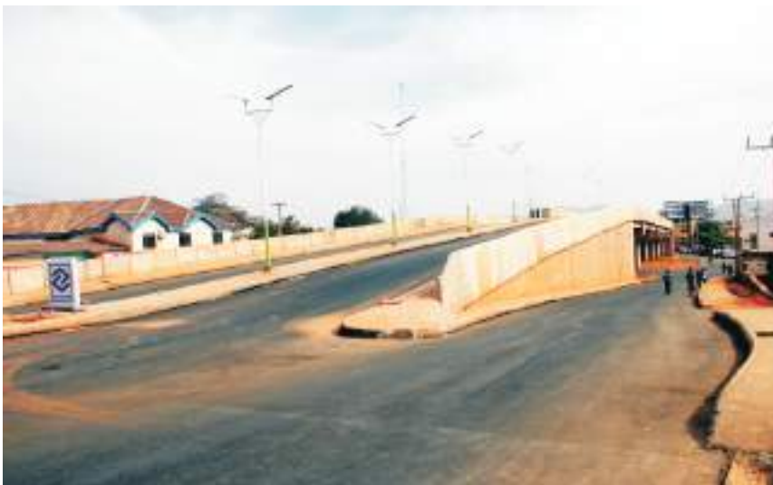
Photo showing the flyover from Dogon Karfe to Terminus and Lamingo road junction roundabout
