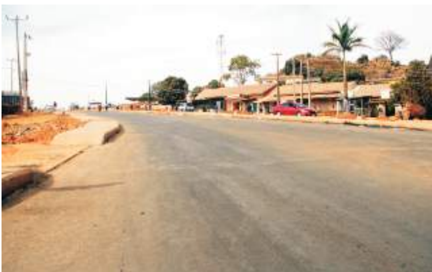
Newly completed road along Lamingo Junction roundabout
