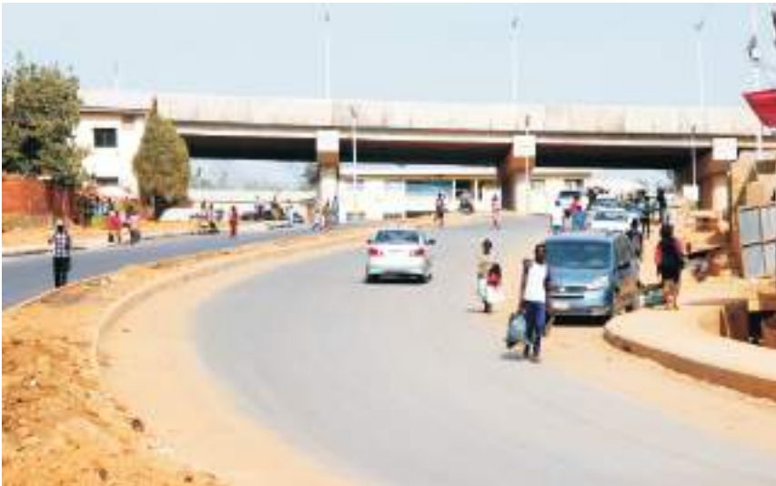
Front view of the flyover
