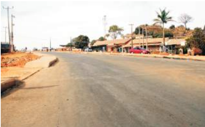
Newly completed road along Lamingo Junction roundabout
