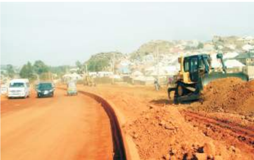
Level of work on the Lamingo Junction roundabout
