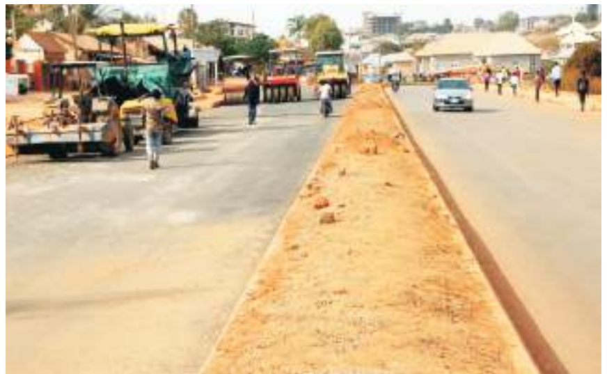
Level of the dualization work in progress as captured yesterday
