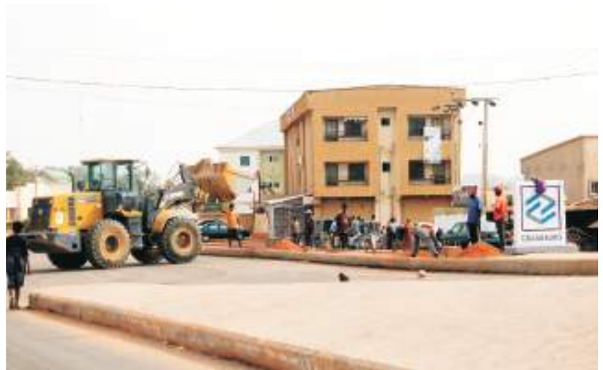
Earth moving equipment putting some finishing touches on the flyover
