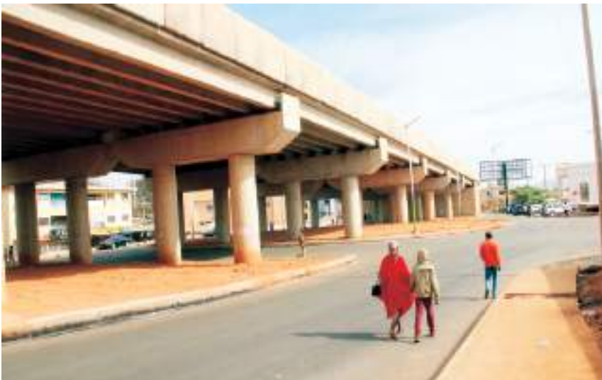
Photo shows the lane from Dogon Karfe to Terminus completed
