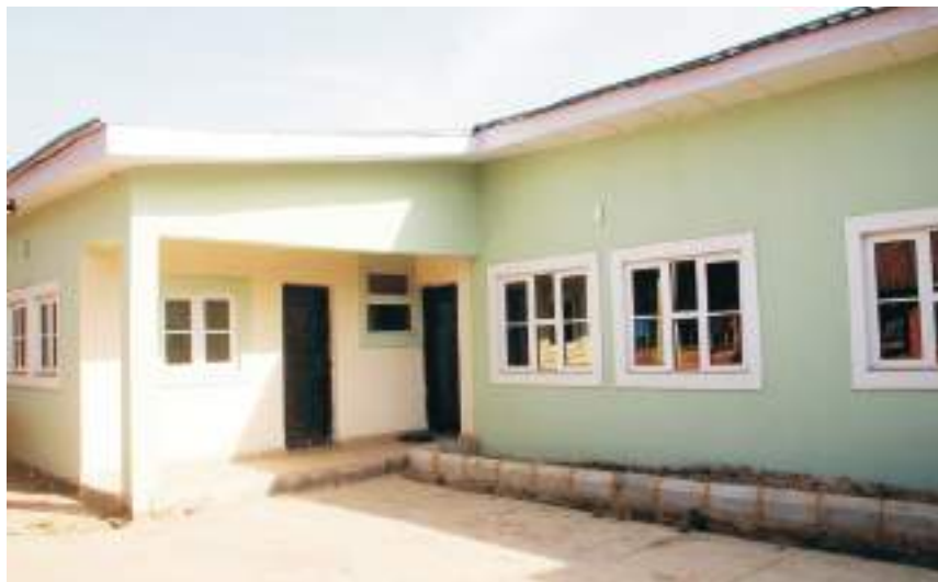
Site of the remodeled NUJ Secretariat inspected by Governor Lalong
