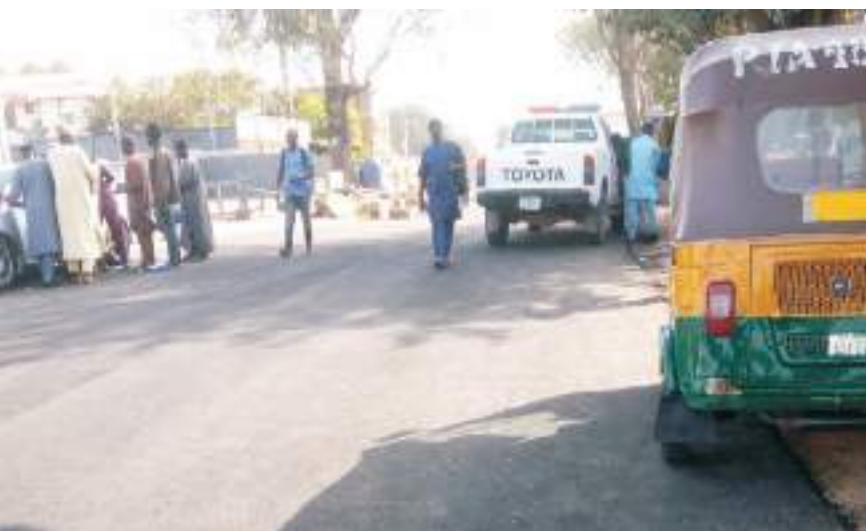
Works in progress at some roads visited
