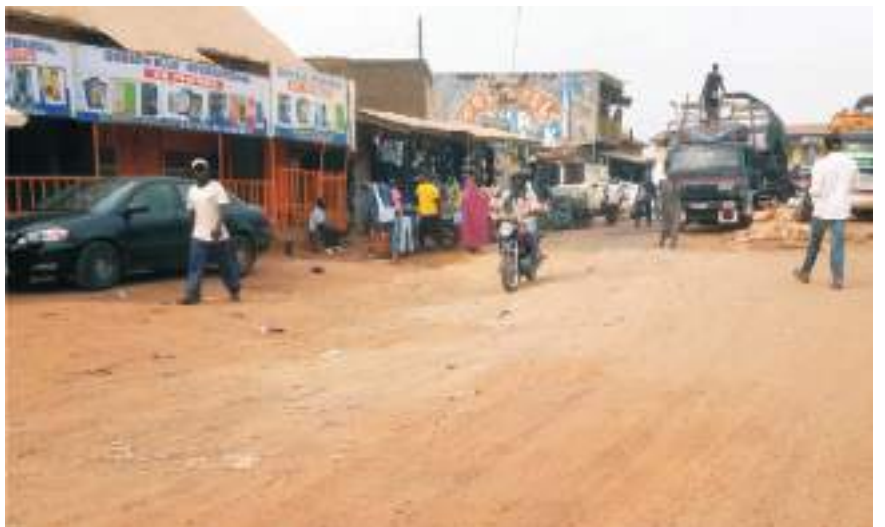
This road from Bauchi Rd junction to Bayan Banki washed out completely
