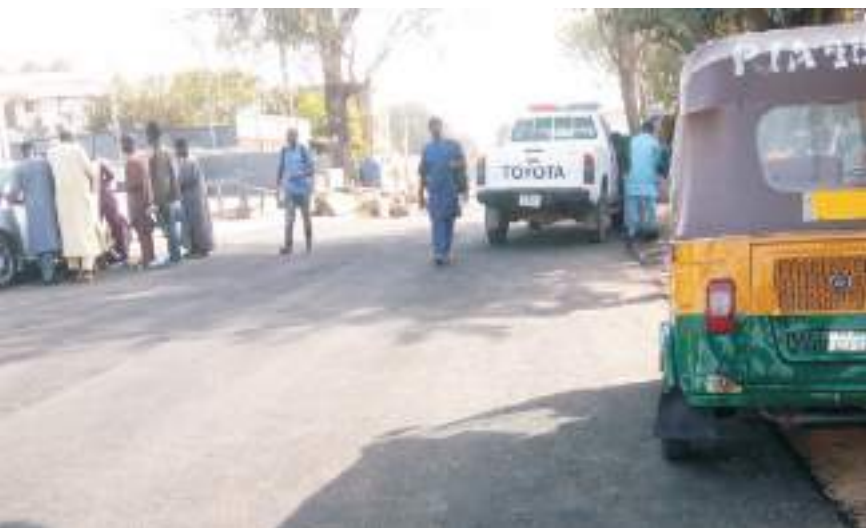
Work in progress at some roads visited
