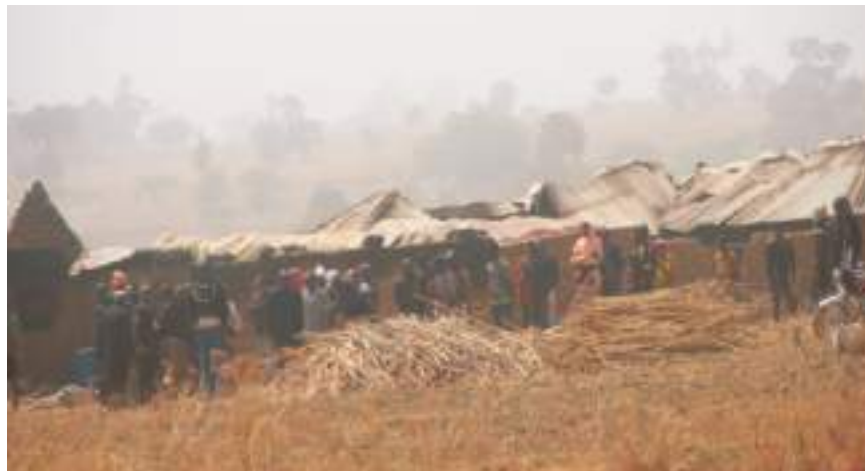
One of the burnt houses inspected by the Governor and entourage
