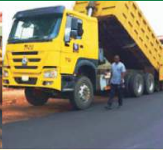
Building Materials-NOUN-Sabon Barki-Bukuru Lowcost Road Network
