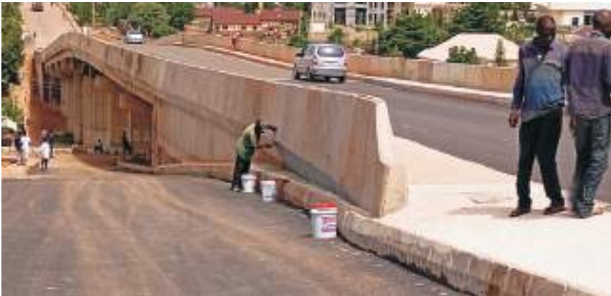
On-going work at the Baba Akila Machunga-Abattoir flyover
